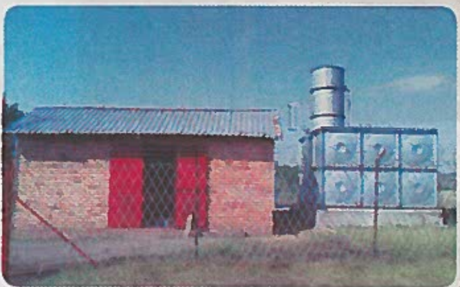
Gomora water purification project
