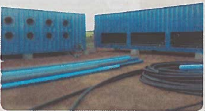
Buffelspruit water purification project
