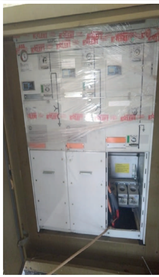
New switchgear being installed at the Driekoppies Dam
